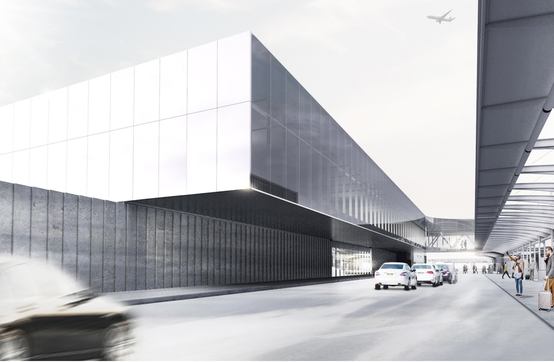
Future REM station at the Montréal-Trudeau International Airport
