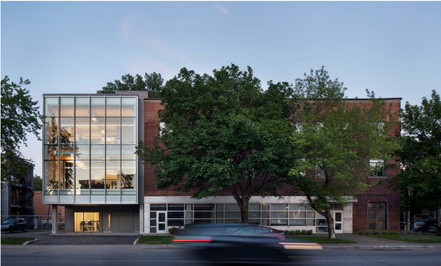
Jodoin Lamarre Pratte architectes' offices © Adrien Williams
